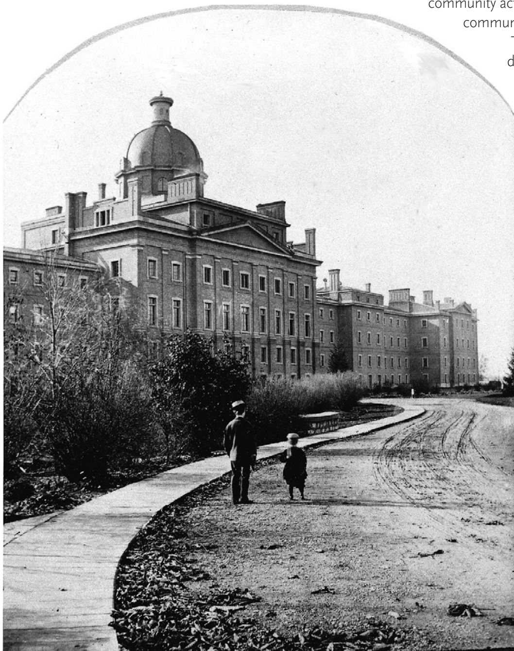
This photo of the 'Provincial Lunatic Asylum' was taken in 1868 by the Notman & Fraser Studio and is provided courtesy of the Toronto Reference Library, Baldwin Room.
